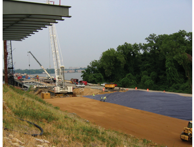
To improve roadway life utilize a nonwoven fabric to separate native soil and aggregate.
