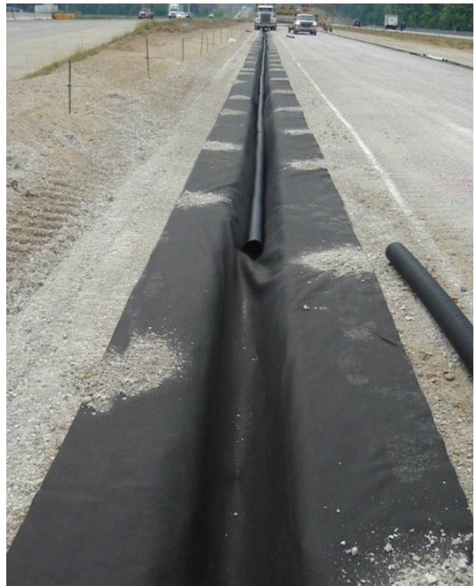
A geotextile used as a trench liner allows water to pass into the pipe, while filtering out soil fines and protecting the pipe from clogs.
