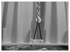
The MC-7200 contains built in ropes at the feet on both sides of the chambers to be used to lift and place the chambers using an excavator. No more than two chambers should be lifted at a time using the ropes. A 14' x Joint" Be sure that the chamber 3/8" (10 mm) chain is recommended along with a 5/8" (16 mm) Jaw and Eye Swivel. Using this method, chambers can be placed directly on an existing row. Using too long of a chain may cause the chambers to be less stable during picking.
