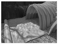
Place a continuous layer of ADS Plus fabric between the foundation stone and the Isolator Row Plus chambers, making sure the fabric lays flat and extends the entire width of the chamber feet. When used on an Isolator Row Plus, a 24" FLAMP (flared end ramp) is attached to the inside of the inlet pipe with a provided threaded rod and bolt. The FLAMP then lays on top of the ADS Plus fabric.
