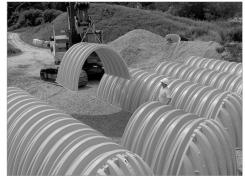
Continue installing chambers by overlapping chamber end corrugations. Chamber joints are labeled "Lower Joint - Overlap Here" and "Build this direction - Upper placement does not exceed the reach of the construction equipment used to place the stone. Maintain minimum 9" (230 mm) spacing between MC-7200 rows.
