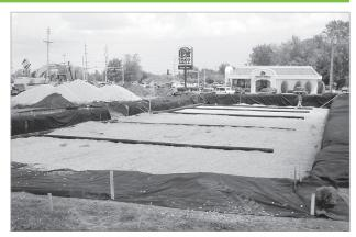
Place clean, crushed, angular stone foundation 9" (230 mm) min. Install underdrains if required. Compact to achieve a flat surface.
