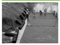
Install manifolds and lay out ADS Plus Fabric at inlet rows. Place ADS Plus Fabric at each inlet end cap parallel to the row (min. 17.5 ft (5.33 m)). Place a continuous piece entire length of Isolator Plus Row(s). Align the first chamber and end cap of each row with inlet pipes. Contractor may choose to postpone stone placement around end chambers and leave ends of rows open for easy inspection of chambers during the backfill process.
