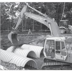
Initial embedment shall be spotted along the centerline of the chamber evenly anchoring the lower portion of the chamber. This is best accomplished with a stone conveyor or excavator reaching along the row.
