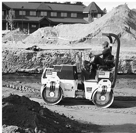
Install non-woven geotextile over stone. Geotextile must overlap 24" (600 mm) where edges meet. Compact at 24" (600 mm) of fill. Roller travel parallel with rows.
