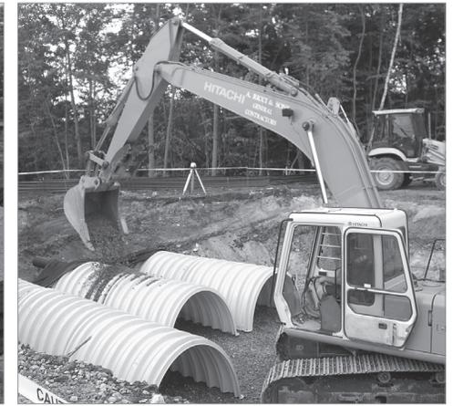
Initial embedment shall be spotted along the centerline of the chamber evenly anchoring the lower portion of the chamber. This is best accomplished with a stone conveyor or excavator reaching along the row.
