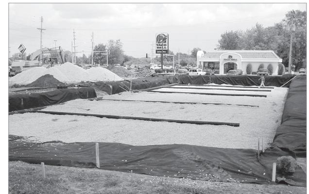
Place clean, crushed, angular stone foundation 9" (230 mm) min. Install underdrains if required. Compact to achieve a flat surface.
