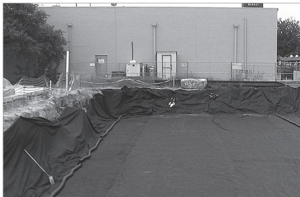
Place non-woven geotextile over prepared soils and up excavation walls.
