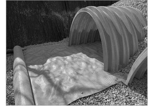
Install manifolds and lay out ADS Plus Fabric at inlet rows. Place ADS Plus Fabric at each inlet end cap parallel to the row (min. 17.5 ft (5.33 m)). Place a continuous piece entire length of Isolator Plus Row(s). Align the first chamber and end cap of each row with inlet pipes. Contractor may choose to postpone stone placement around end chambers and leave ends of rows open for easy inspection of chambers during the backfill process.
