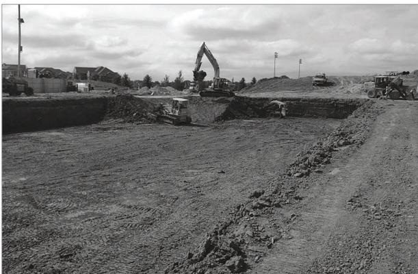
Excavate bed and prepare subgrade per engineer's plans. Plans and specifications should include Best Management Practices (BMPs) to deter contamination of open pits during construction.
