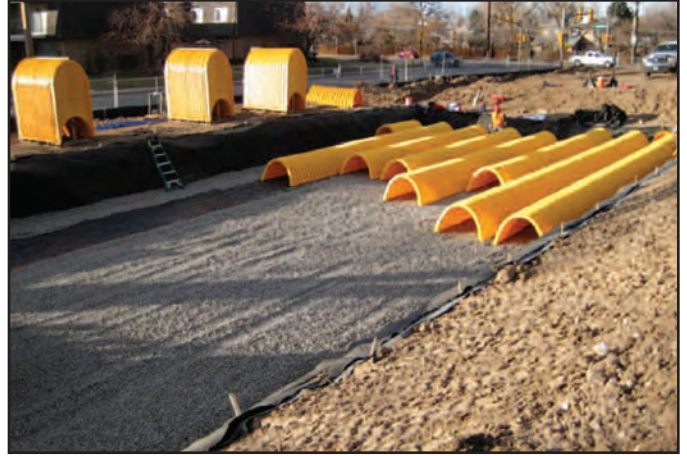
StormTech's system allows basins to be sized to fit specific areas. At SouthGlenn, there are six separate basins.
