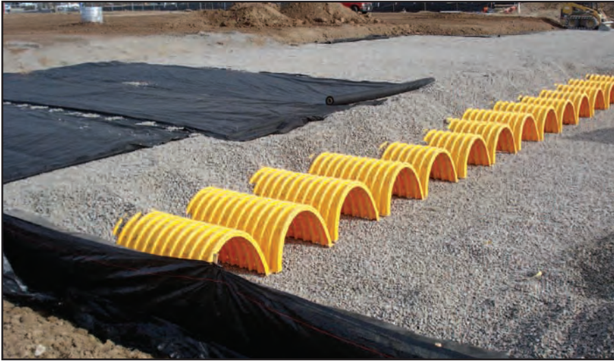
Non-woven filtering geotextile is placed over the rock-covered chambers, allowing water into the basin but not sediment. Nyloplast drain basin, right, will be capped with a ductile iron grate to create an inlet.
