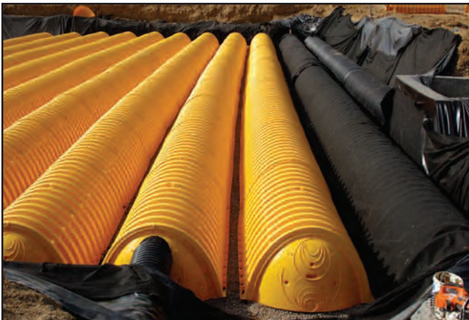
Isolator rows can be seen in these pictures of two different basins. Low flows, including the first flush, are forced into the Isolator Row, which traps sediment as flows to the basin pass through its fabric. Black HDPE pipe seen at left connects to chamber end cap to allow heaviest flows to bypass the Isolator Row and relieve inlet backup. Corrugated metal is set to block the rock so that a light pole and its base can be installed after the parking lot is paved, background at right.
