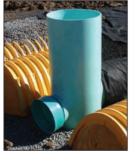
Non-woven filtering geotextile is placed over the rock-covered chambers, allowing water into the basin but not sediment. Nyloplast drain basin, right, will be capped with a ductile iron grate to create an inlet.
