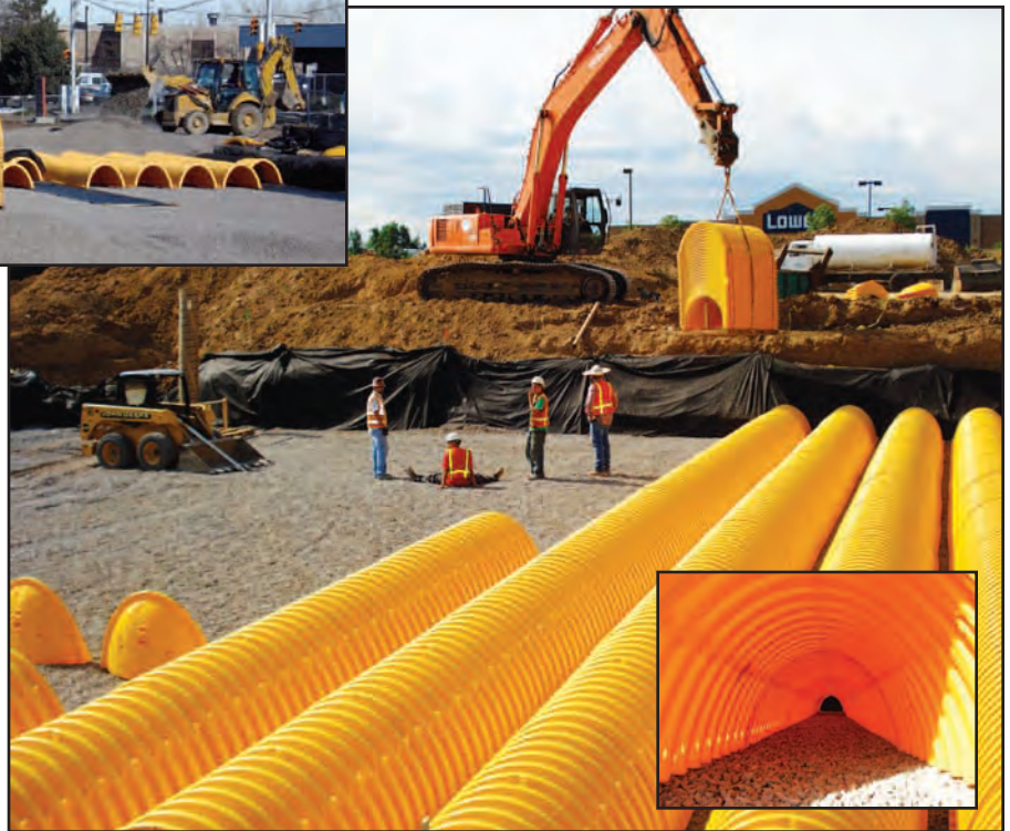
Chamber installation is a quick and easy one-at-a-time process.
