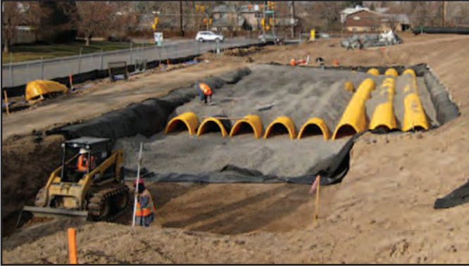
StormTech's system allows basins to be sized to fit specific areas. At SouthGlenn, there are six separate basins.
