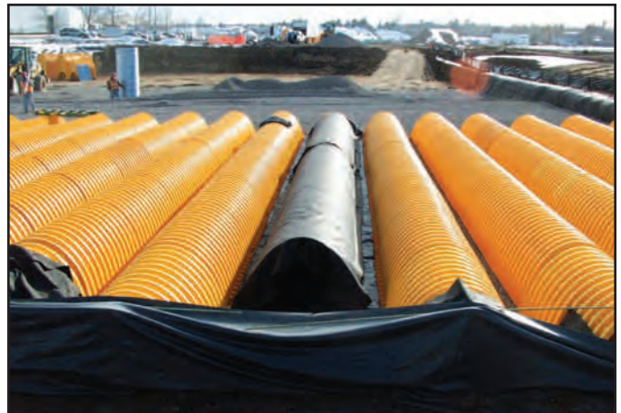
Isolator rows can be seen in these pictures of two different basins. Low flows, including the first flush, are forced into the Isolator Row, which traps sediment as flows to the basin pass through its fabric. Black HDPE pipe seen at left connects to chamber end cap to allow heaviest flows to bypass the Isolator Row and relieve inlet backup. Corrugated metal is set to block the rock so that a light pole and its base can be installed after the parking lot is paved, background at right.
