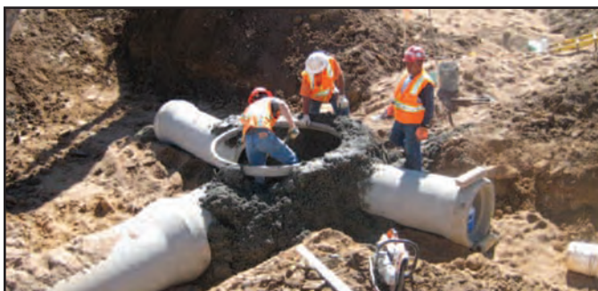
AUI crews set manhole at The Streets At SouthGlenn. At right, SEMSWA Inspector Amber Law checks sediment build-up at one of the site’s temporary detention ponds for erosion control during construction.
