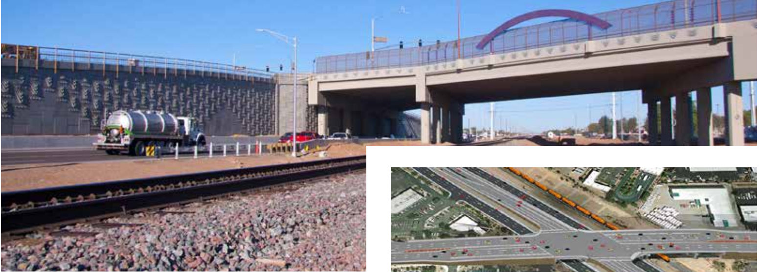
The new interchange is a median urban diamond design (see inset photo), with traffic now diverted over the railroad tracks.
