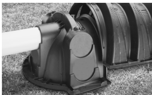
3. Place first chamber onto endcap.
