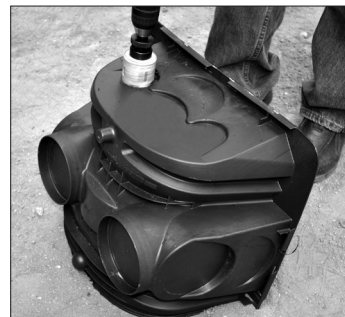
2. Drill pressure pipe hole.
