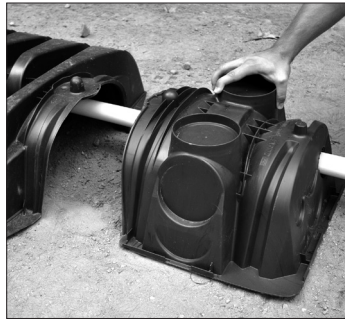
11. Lateral pipe through endcap.
