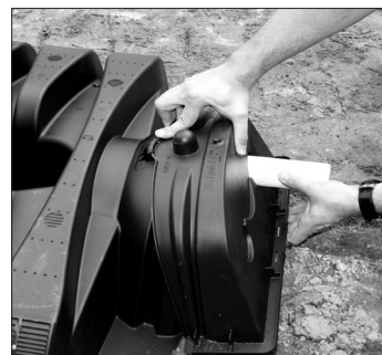
4. Place endcap over inlet end.
