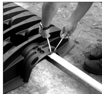
5. Secure pressure pipe.
