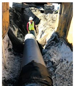
the Florida Department of Transportation (FDOT) 2014 Standard Specifications for Road and Bridge Construction, Section 948-7. The FDOT standard has been revised to include 100-year design service life pursuant to AAS-HTO M330. The pipe is typically used for side drain, cross drain and storm sewer projects.
