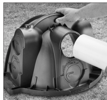
5. Insert inlet pipe.
