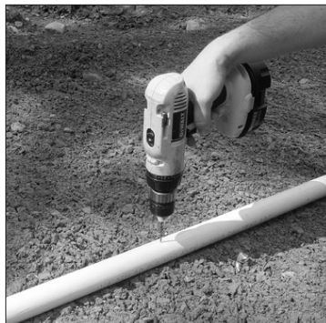
1. Drill hole in pipe.
