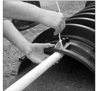
5. Secure pipe to chamber.
