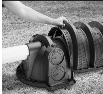
3. Place first chamber onto endcap.
