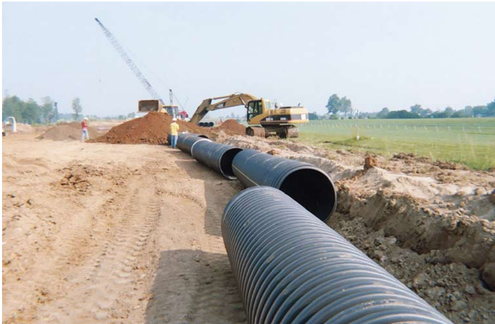
Elevating the grandstand apron required an end-to-end drainage structure to empty the runoff of the trench and roof drains.
