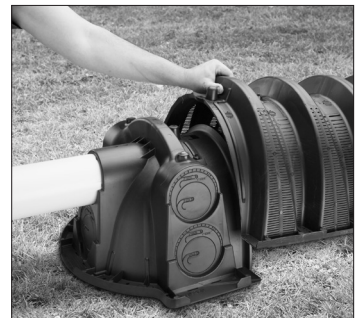
3. Place first chamber onto endcap.
