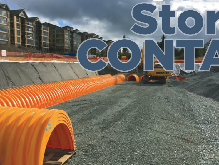
The modular arch chamber system is made up of over 3,300 segments able to retain over 21 million liters.
