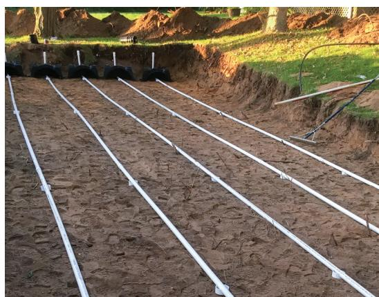
The project site encompasses two acres but a large portion of the property is wooded and the homeowner wanted to preserve as many trees as possible. Access was tight so the Infiltrators chambers enabled the team to complete the installation with a small excavator. Only a limited number of small shrubs were moved and then replanted in the same location after the installation was complete.
