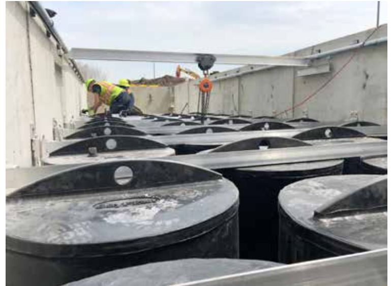
To meet New Jersey Department of Environmental Protection requirements, 109 BayFilter units were used to create the stormwater filtration system at the old Harrison Avenue landfill in Kearny.
