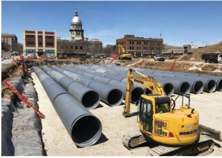
The underground detention facility is comprised of a 2,300-foot network of five-foot diameter pipes constructed in an 11-foot-deep excavation, and designed to hold 340,000 gallons of stormwater at maximum capacity. The entire system was wrapped with a geosynthetic clay liner to protect the pipes from contaminated soils and groundwater, a unique application for a
