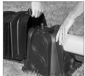
3. Place first chamber onto endcap.
