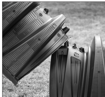
4. Connect the chambers.
