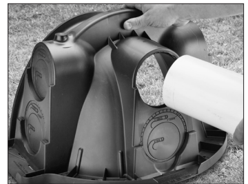
5. Insert inlet pipe.
