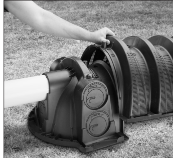
3. Place first chamber onto endcap.
