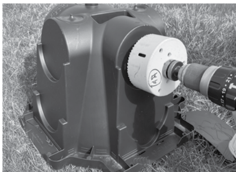
2. Drill the hole on the endcap.
