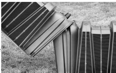
8. Attach endcap to chamber.
