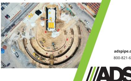
adspipe.com 800-821-6710 Originally, the detention system was specified to be corrugated metal pipe (CMP). The pipe system was flipped to StormTech. N-12 and Nyloplast were on the original plans allowing for ADS to completely supply the park's drainage system with its wide product array.
