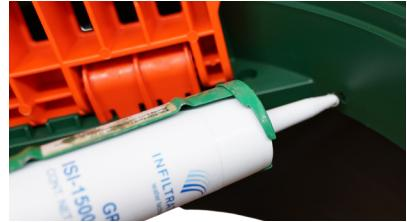
**7.** Reduce the torque and speed of your drill driver and screw (4) #14 2" stainless steel screws into the pilot holes that have been filled with sealant. Tighten these screws in an alternating pattern, just as you would on a vehicle's tire, to prevent the Guardian shifting too much in one direction. Each screw should be tightened over the course of at least 3 intervals (see image in step 5). These screws are included with the Guardian.
