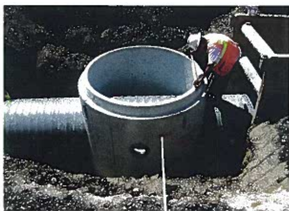
Polypropylene is highly resistant to the hydrogen sulfide gas found in sewers.
