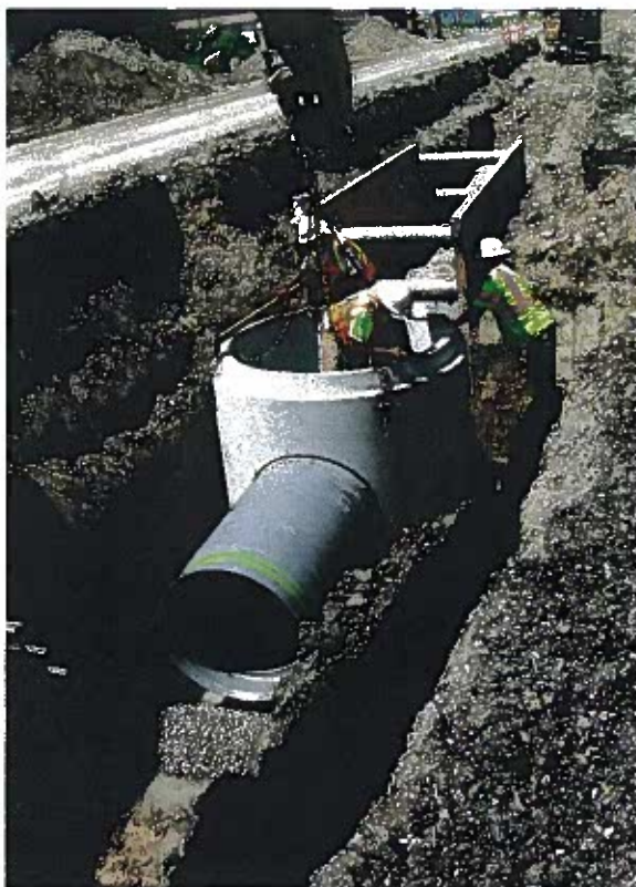
Overall project depth measured 10 to 12 ft and was completed in eight weeks.
