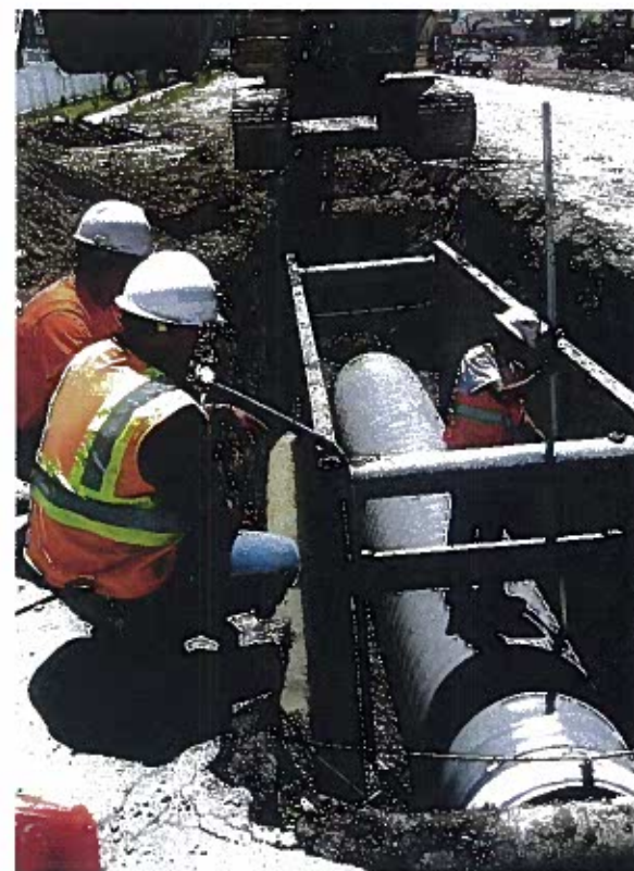
The existing 18-in. trunk line was upgraded to 36-in. pipe, and the existing 36-in. line to 48-in. pipe to accommodate the city's build-out projections.
