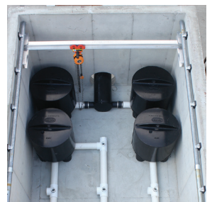
Vault Internal Assembly
