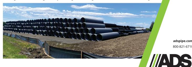
Stormwater from the project site and along County Road 99 was conveyed to nearby creeks by using nearly 16,000' (4,877 m) of N-12 and HP Storm pipe. The stormwater conveyance ran approximately 1.5 miles along County Road 99.
