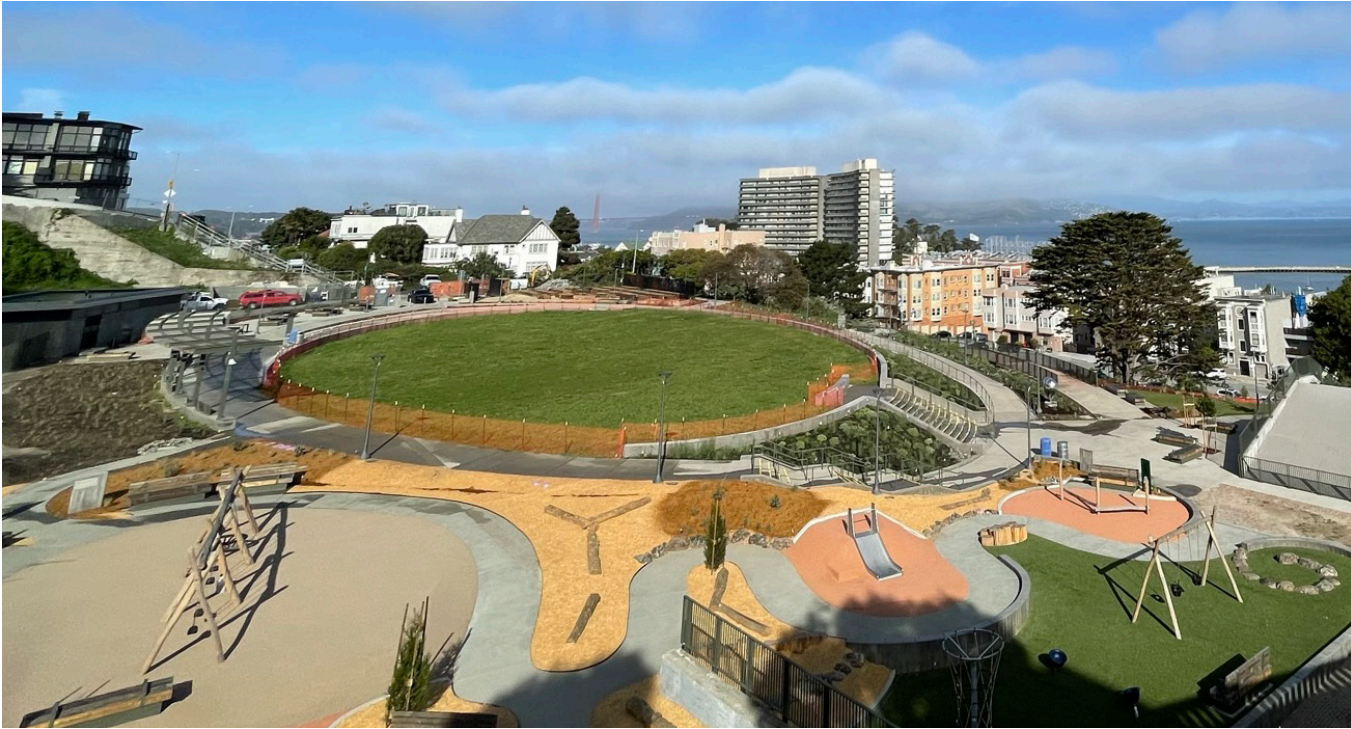
Francisco Park, San Francisco, Ca; (Front cover: StormTech Chambers being installed at Francisco Park).
