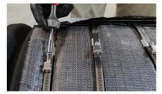
**Step 2:** Make sure that the center strap is in the butt joint groove and that the outside straps are on each side of the joint between the corrugations. Tighten the straps with the proper tools, starting with outside strap.
