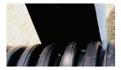
**Step 1:** Clean the external portion of the joint to ensure that foreign materials do not interfere with direct contact between the mastic sealer and the joint to be sealed.
