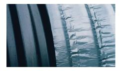
**Step 3:** Remove the protective film from the closing flap and cover the exposed portion of the strap, completing the joint.
