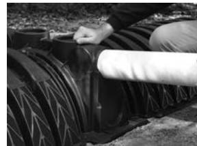
6. Insert connection pipe.
