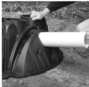
5. Insert inlet pipe.
