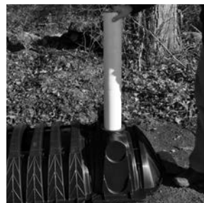
2. Pipe in endcap inspection port.
