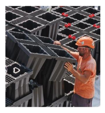
The Aquabox Cube has a central opening which enables a 300 mm (12") N-12 riser pipe to reach the surface. A Nyloplast inline drain finishes the top of the riser pipe.
