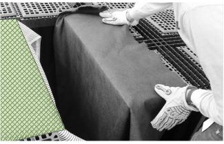
For Isolator Rows that end within the bed, install the module outside the end of the row with a side panel facing the Isolator Row. Place a piece of ADS 601 geotextile between the Isolator Row and this final module.
