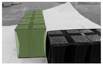
Fold the upper layer of ADS Plus geotextile back over the previously installed modules. Then install the modules of the Isolator Row.
