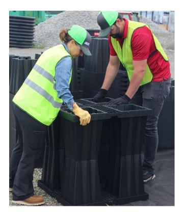
During installation, it is possible to walk on top of the modules. It is forbidden for operating machines, even small ones, to pass over the structure without proper covering.
