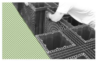
As the next row of modules are assembled, install side panels on the module sides facing the Isolator Row. No joints are used between the Isolator Row and abutting row modules
