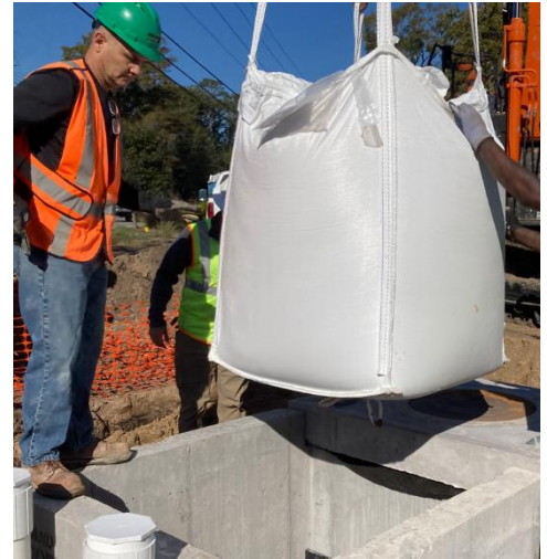
Figure 15: Filtration media bag, installing filter media
