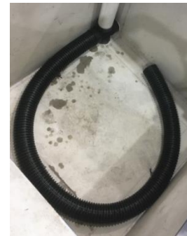
Figure 4: Example underdrain placement
