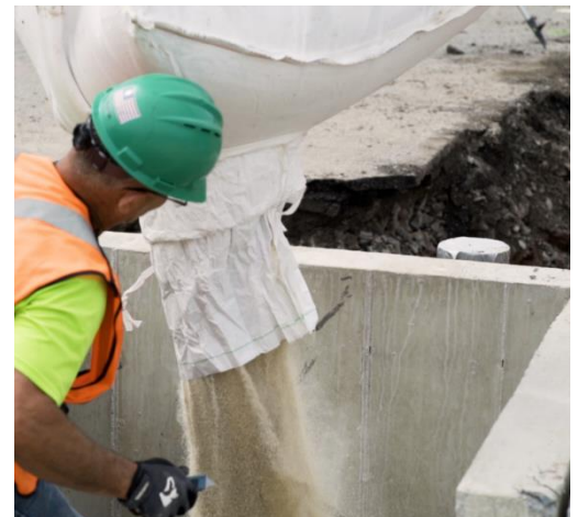
Figure 16: Filtration media bag, installing filter media
