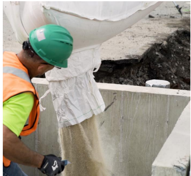
Figure 16: Filtration media bag, installing filter
