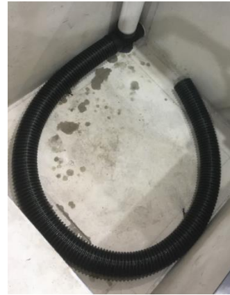
Figure 4: Example underdrain placement
