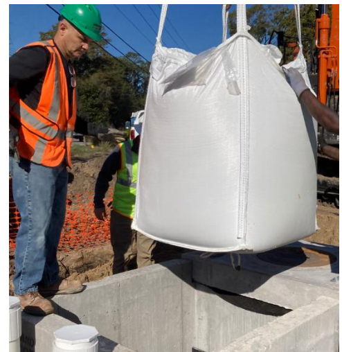
Figure 15: Filtration media bag, installing filter media
