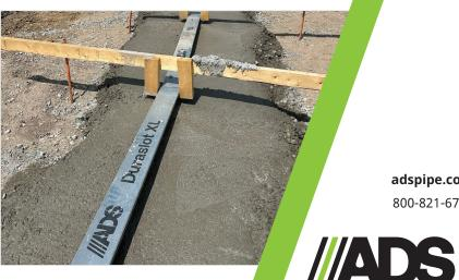
adspipe.com 800-821-6710 fastened together with normal Duraslot XL couplers with a maximum gap of ¼" (6 mm).
