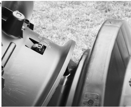
7. Attach endcap to chamber.
