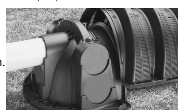
4. Insert inlet pipe.
