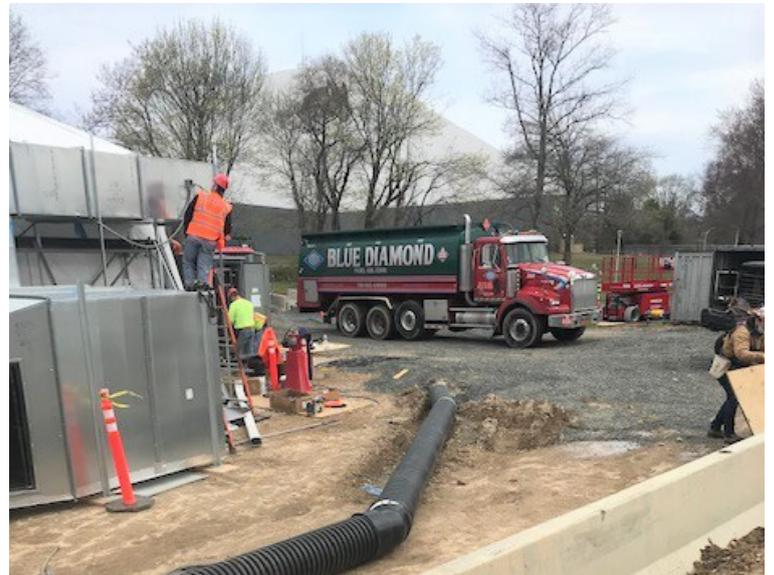
The ADS N-12 stormwater drainage pipe was run under roads and parking areas at the U.S. Army Corps of Engineers’ Long Island, New York field hospitals.
