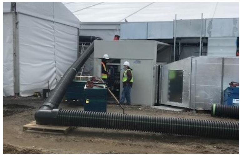
Rain water is conveyed from the roof to gutters then to ADS N-12 pipe where it drains into swells.
