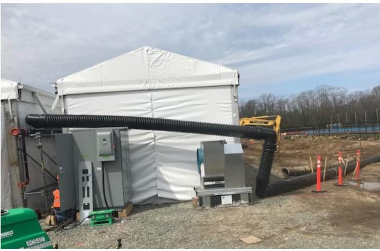
ADS N-12 pipe was used to convey rain water from the roofs of the field hospitals at Stony Brook and SUNY Old Westbury, New York.
