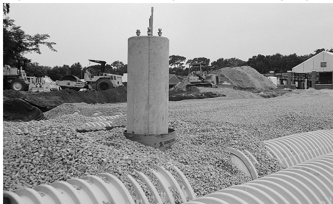
Figure 13 – Chamber bed placed around light post.
