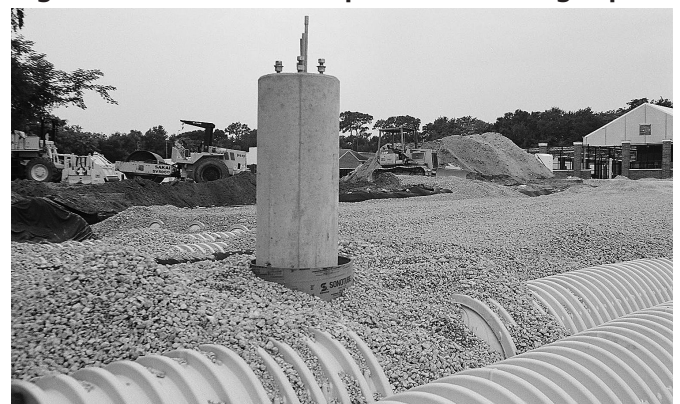
Figure 13 - Chamber bed placed around light post.
