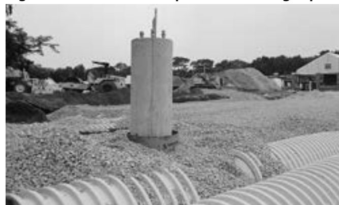
Figure 13 - Chamber bed placed around light post.
