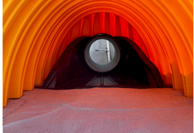
Looking down the Isolator Row PLUS
