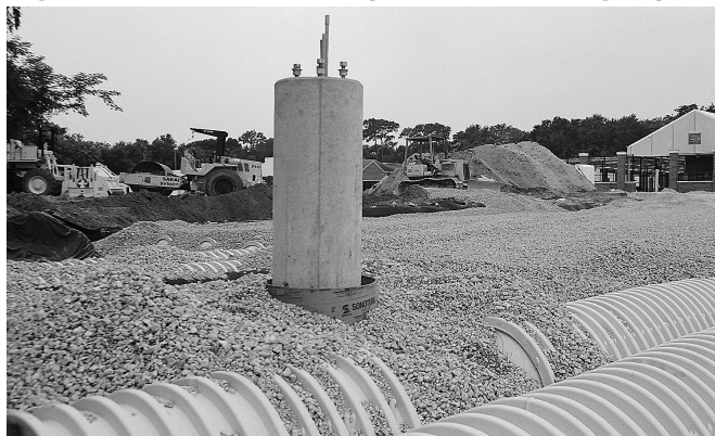
Figure 13 - Chamber bed placed around light post.
