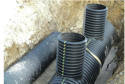
N-12 Rainwater Harvesting
