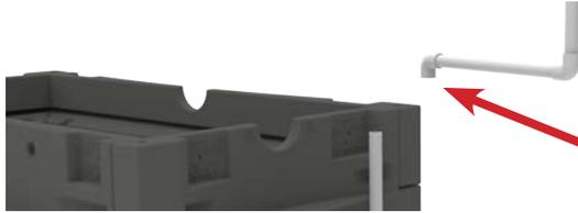
Place the Air Lift Assembly in the tank through the outlet end port. Ensure the Air Lift Assembly is placed on the floor of the tank and is not sitting on top of a rib. The elbow connected to the bottom of the Air Lift Assembly must be directed toward the ECOPOD reactor box.
