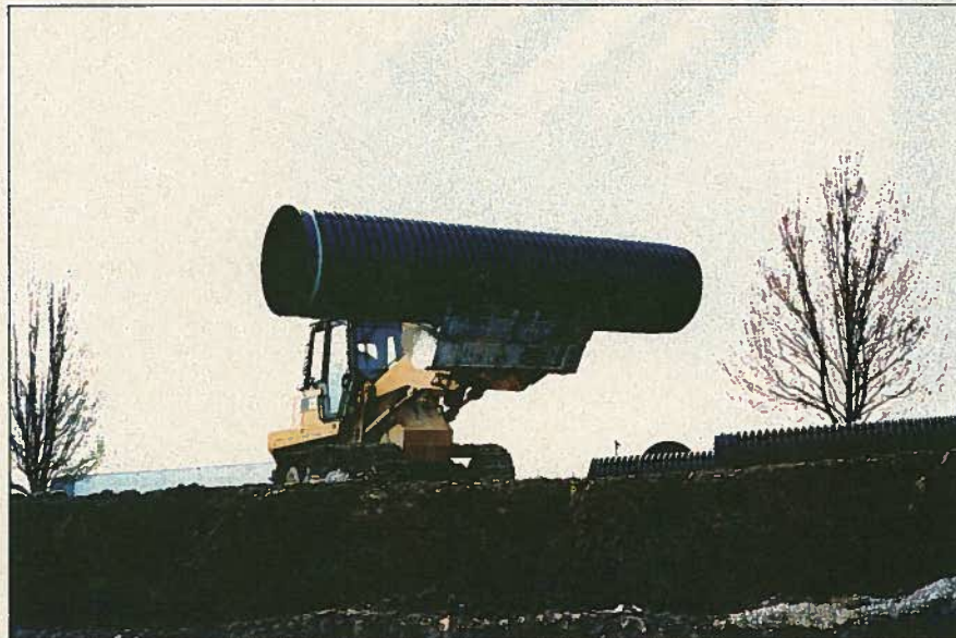
Researchers at Drexel University have found through the development of a new test protocol that the life expectancy of HDPE pipe surpasses the estimated 20- to 100-year service life.
