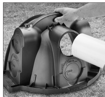
5. Insert inlet pipe.
