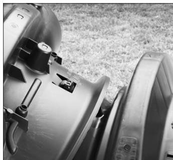
8. Attach endcap to chamber.
