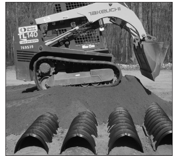
3. Push sand between and over the chambers.
