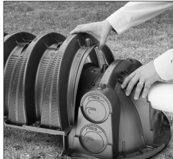
3. Place first chamber over endcap.
