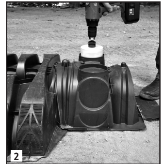
Drill top of Quick4 Plus All-in-One 8 Endcap.
