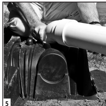
Insert inlet pipe.
