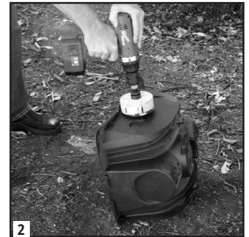
Drill bottom of endcap.
