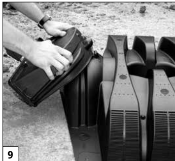
Place end cap outlet end.
