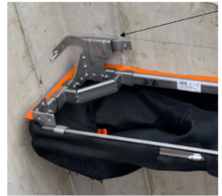
Figure 3: FlexStorm filters bolted to wall
