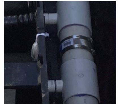
Figure 8: Thin Pipe Coupler
