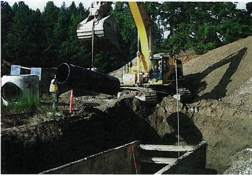
Hancor HDPE pipe is designed for sanitary sewer systems, which are usually buried deeper and subject to greater water pressure than corrugated HDPE pipe used for storm sewer installations.
