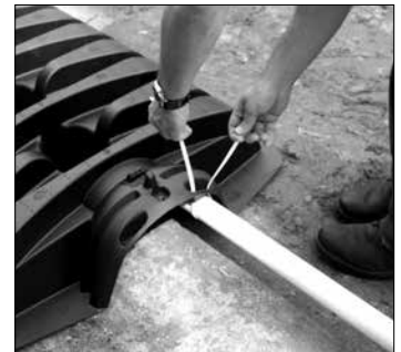
4. Place endcap over inlet end.
