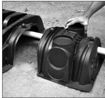
11. Lateral pipe through endcap.
