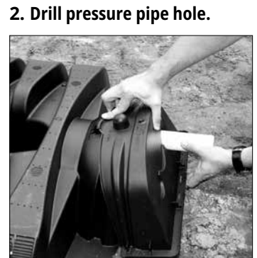
2. Drill pressure pipe hole.
