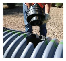
Use the coupon to estimate the separation between the two sleeves and fit the two sleeves together. Be sure the gold lines on the sleeves are lined up.
