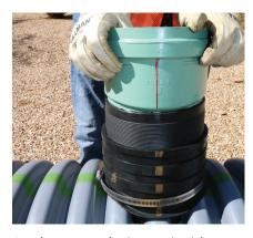
Apply soap solution to inside of the inner sleeve and on the PVC hub. Insert the PVC hub into the sleeve by hand until snug fit, aligning the red line on the hub with the gold lines on the rubber sleeves.
