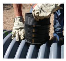
Insert the rubber sleeves into the cored hole, with the gold lines perpendicular to the pipe. Once in place, pull up on the inner sleeve and push down on the outer sleeve until fitted to the host pipe.
