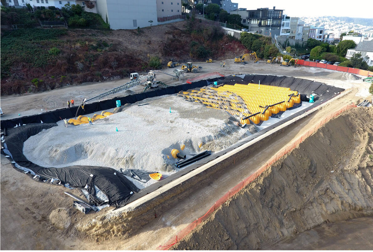
Left: A rain capture system in Francisco Park in the Russian Hill area is being installed.
