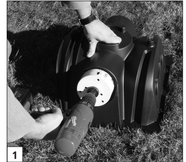
Drill endcap on side or top.
