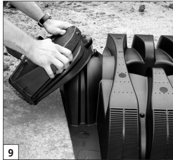
Place end cap outlet end.
