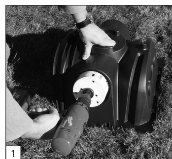
Drill endcap on side or top.
