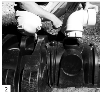
Insert Quick4 Plus Periscope.
