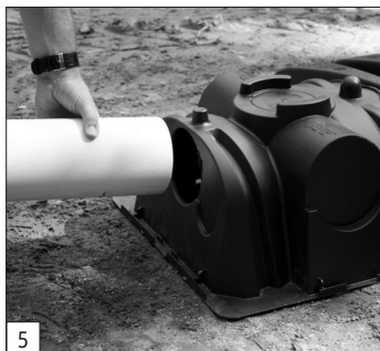
Insert inlet pipe.
