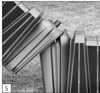
Connect the chambers.
