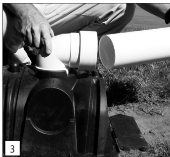
Connect inlet pipe.
