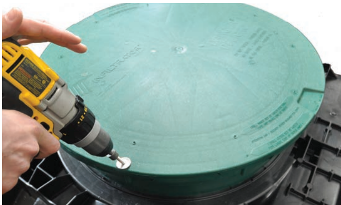
Fasten the lid to the riser with screws provided.
