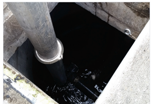
Jet Vactoring Through Access Hatch
