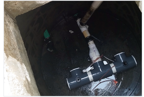
Manifold Tee View of a Cleaned System
