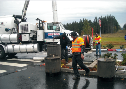
BayFilter System Cleanout
