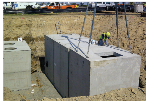
Vault End Section
